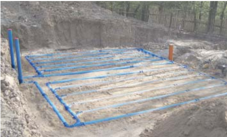
Figur 4. REHAU system AWADUKT Thermo.
